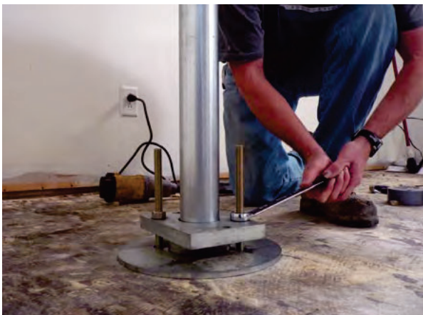
Figure 2.71 Slab pier drive adaptor installed
