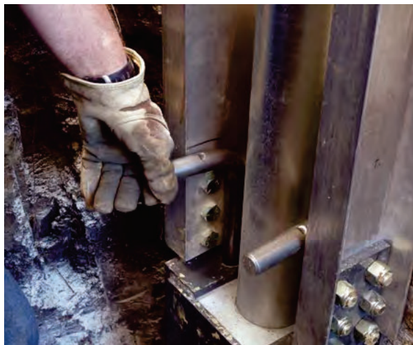
Figure 2.28 PP288 drive stand secured to the bracket with L-pins
