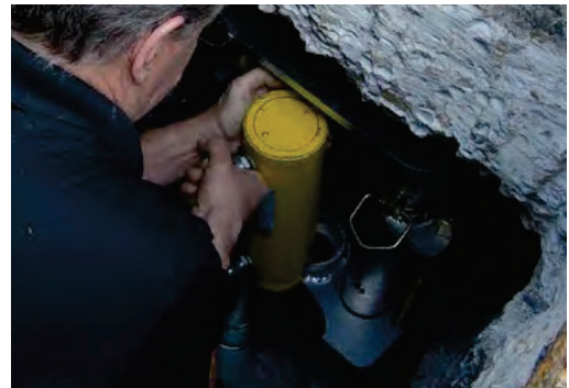
Figure 2.51 Placement of hydraulic drive cylinder
