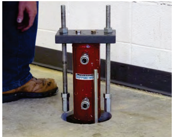
Figure 2.76 Lift cylinder assembly set on pier cap
