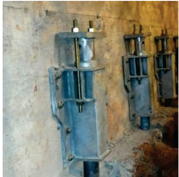
Figure 2.46 Flush-mount bracket installation
