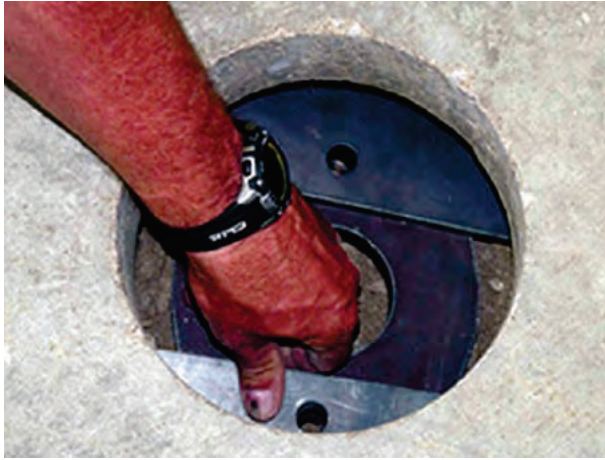
Figure 2.68 Main plate and wing plates positioned and aligned beneath the slab
