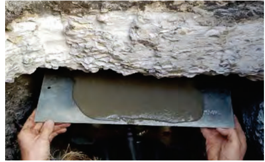
Figure 2.49 Grout plate used to create uniform bearing
