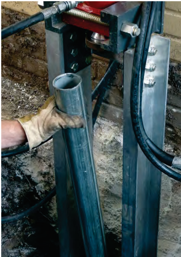
Figure 2.34 Installing PP288 push pier tube
