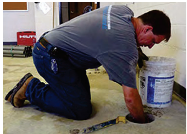
Figure 2.67 Excavating beneath the slab
