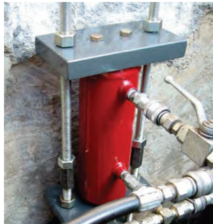
Figure 2.12 Foundation Supportworks FS35LCA lift cylinder assembly
