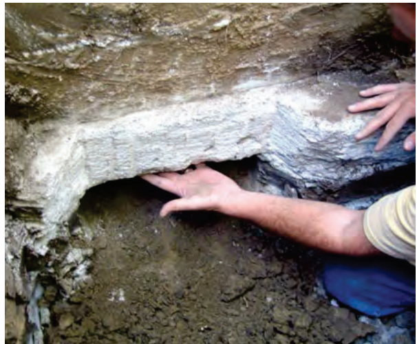
Figure 2.21 Checking underside of footing for proper preparation
