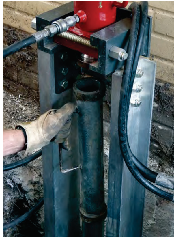
Figure 2.35 Driving tube tool set in place for second stage of push
