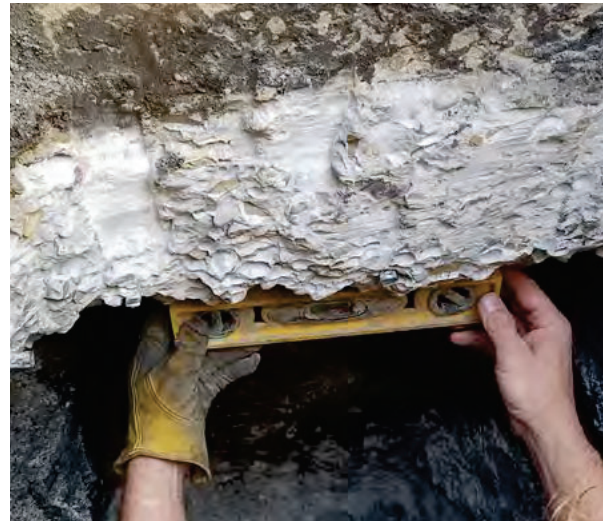
Figure 2.48 Prepare bottom of footing with chipping hammer, as necessary, to create a flat and level surface
