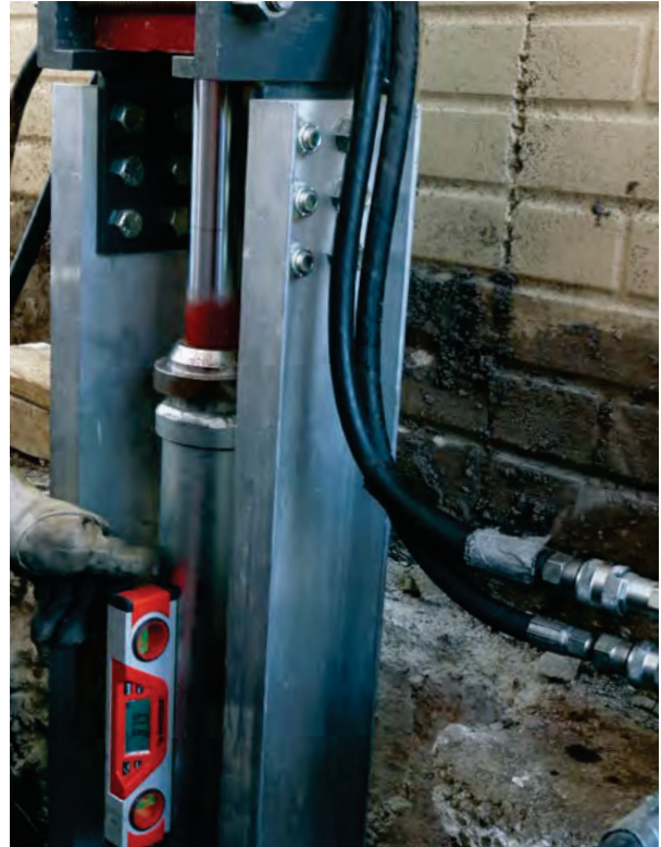
Figure 2.32 Checking drive stand alignment with digital level
