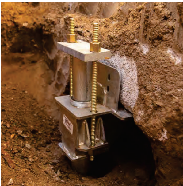
Figure 2.39 PP288 bracket ready for lift cylinder assembly
