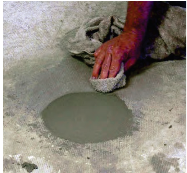
Figure 2.83 Finishing concrete
