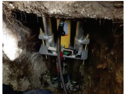
Figure 2.52 Extend hydraulic cylinder to engage footing
