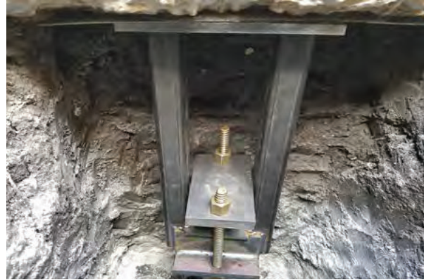
Figure 2.58 Completed concentric pier installation
