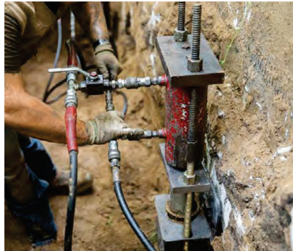
Figure 2.40 Connection of lift cylinder assembly
