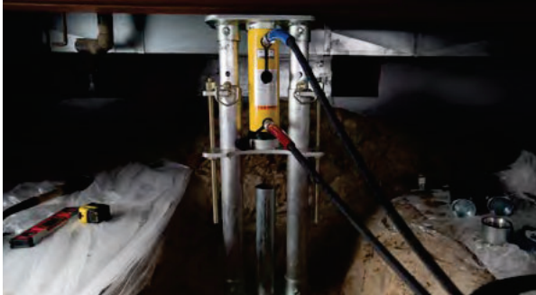
Figure 2.60 Concentric pier drive stand beneath main girder in crawl space
