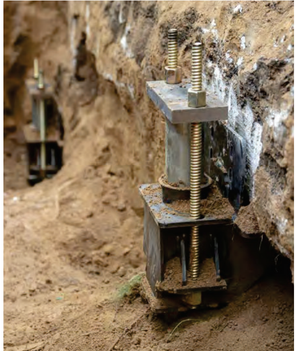
Figure 2.42 System locked off; pier installation complete
