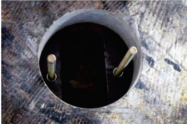
Figure 2.69 Threaded rods installed
