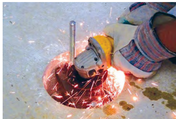
Figure 2.81 Cutting the threaded rods
