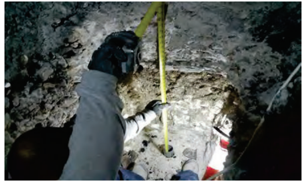
Figure 2.54 Measure from bottom of footing to top of installed pier section
