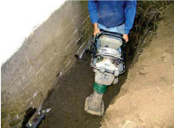
Figure 2.44 Backfill excavations and compact soil
