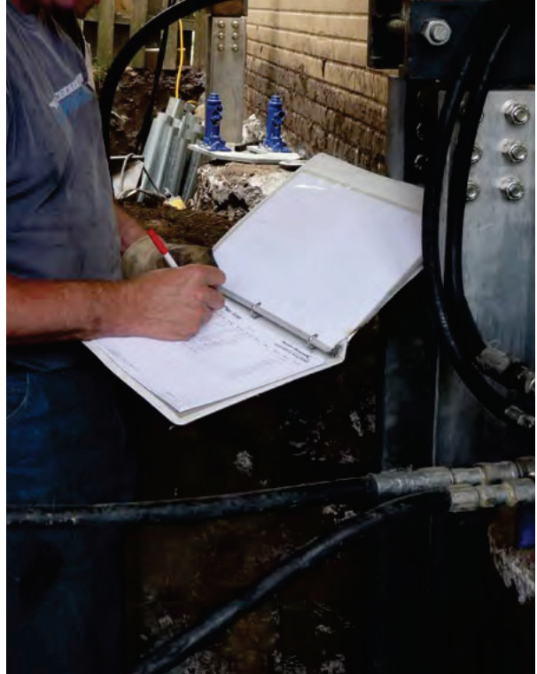
Figure 2.36 Pressure readings are recorded for each pier tube
