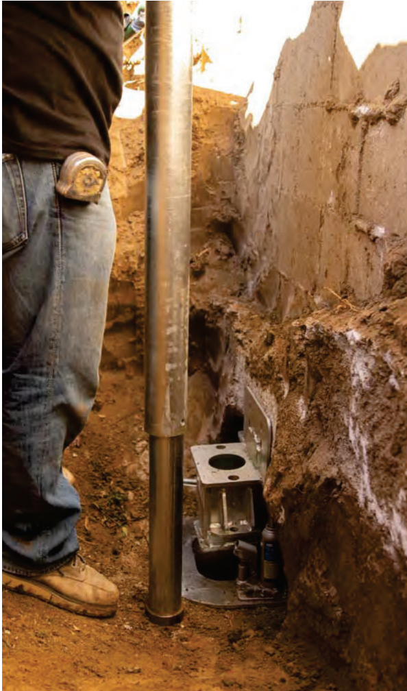
Figure 2.25 Exterior sleeve slid over the starter tube
