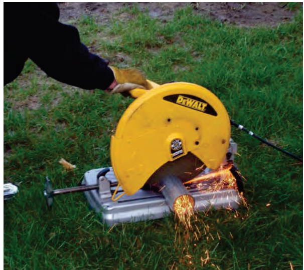
Figure 2.37 Cutting pier tube to desired length with a chop saw
