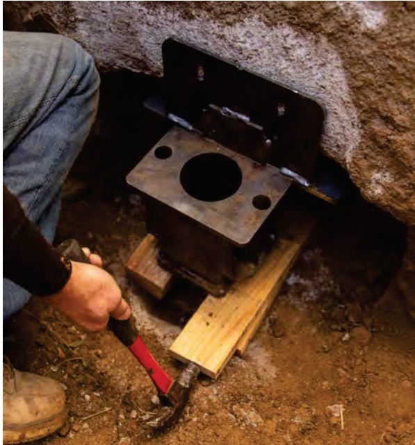
Figure 2.23 Temporary bracket support with wood cribbing
