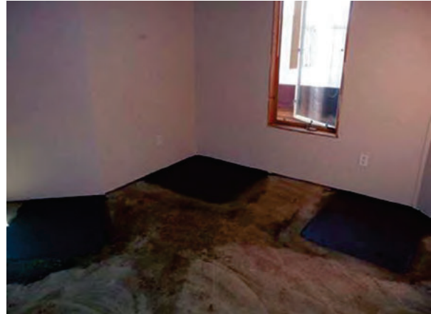
Figure 2.45 Concrete placement at interior pier locations
