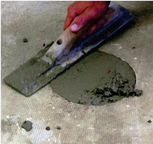
Figure 2.82 Patching holes at pier locations
