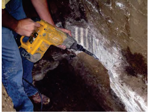
Figure 2.20 Smoothing the vertical and horizontal bearing surfaces with a chipping hammer
