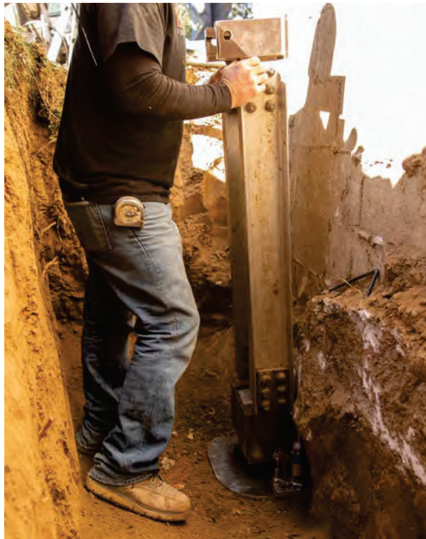
Figure 2.27 Drive stand for PP288 push pier system fitted to the bracket
