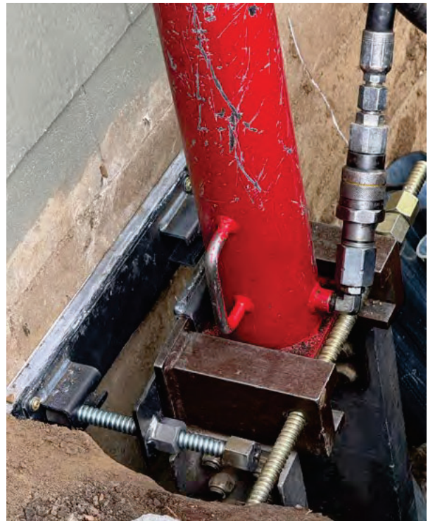
Figure 2.33 Adjustable cribbing tool used to set installation angle
